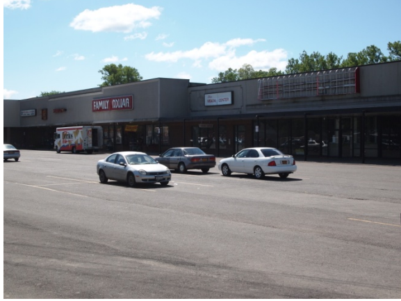
Cedar Street Mall, a retail development with mixed-use potential.
