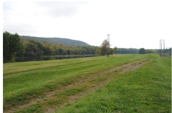
View from the levee of the Chemung River near Fisher Street.
