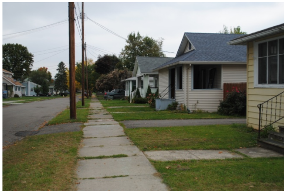
Some of the homes on this side of the street are in need of maintenance, as well as sidewalk repairs and street trees.
