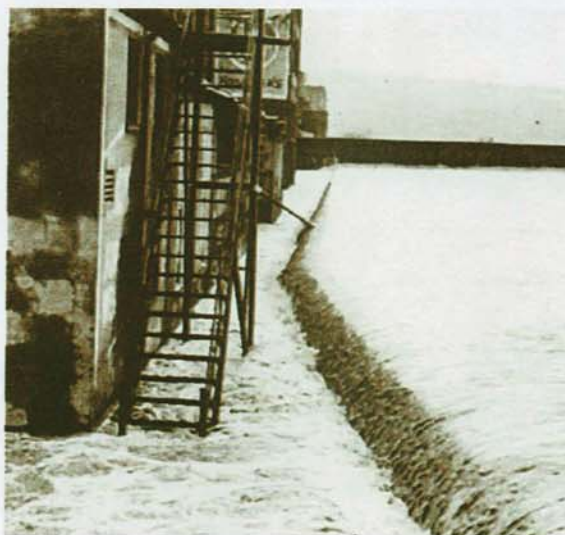
The 1972 Tropical Storm Agnes flood overtopped the floodwall in Elmira and other levees.
